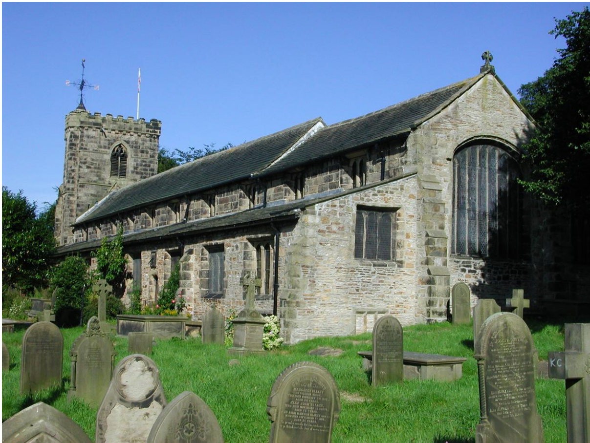
Exterior of Kildwick Church, showing the south side of the building. The clear “break” in the roof-line indicates the start of the Tudor extension.
